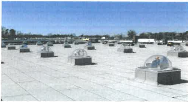
Solar tracking skylights were installed to provide natural light to the dark interiors located in the center of the building.
