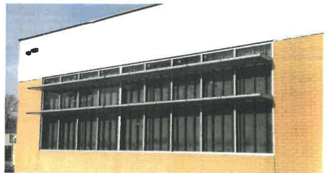
An automated shading system predicts the sun's position to maximize natural light and conserve energy.
