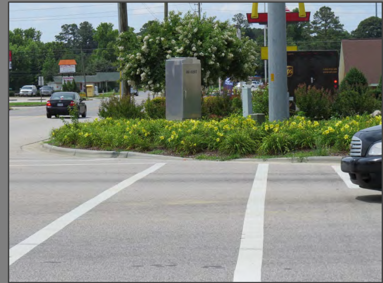
Figure 2-6: Pedestrian curb ramp that was planted with landscaping presents a barrier at NC 55 & 210.
